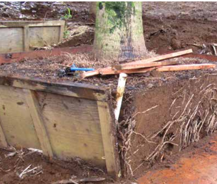
Bismarck palm root ball after 2 years of recovery in a plywood box. The plywood is rated for ground contact and the inside surface is treated with a water sealing compound.
