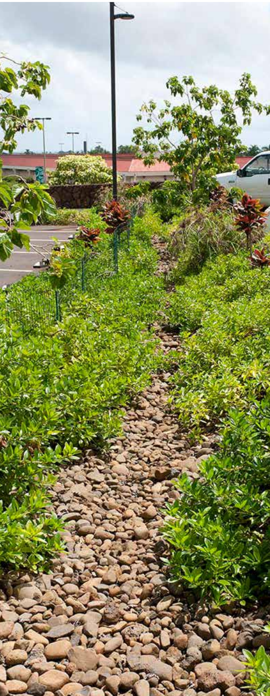
Vegetated bio-filter treats parking lot runoff. Photo Credit: City and County of Honolulu
